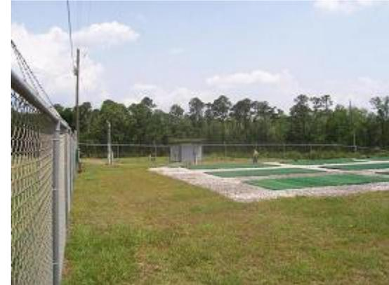
Figure 1 A 30,000 gpd WWTTP (6 of 9 pods visible); control panel in background
