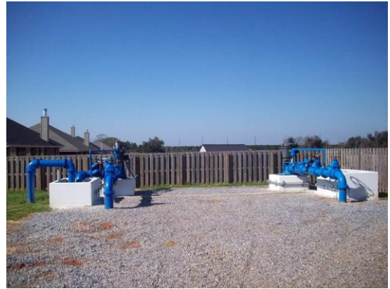
B: Facility's backyard with two wells 41 feet apart
