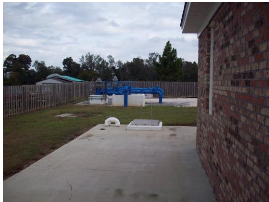
A: West side of plant showing clearwell and wells
