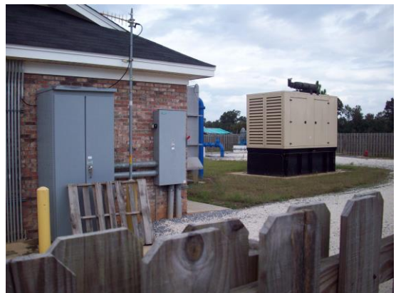
D: East side of plant showing emergency power unit
