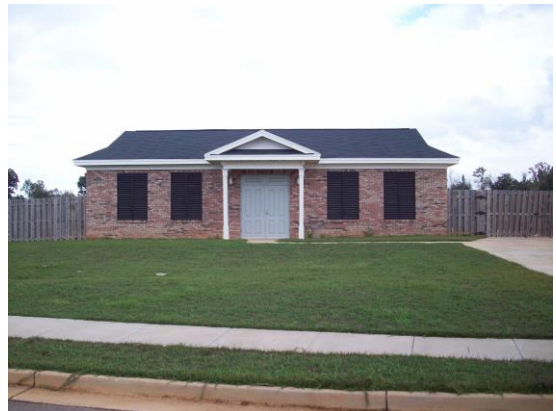
C: Street view of Treatment Plant
